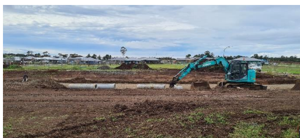
Photograph 4: From near BH1505 (Lot 1507), facing east.
