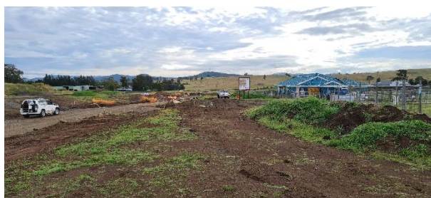
Photograph 2: From near BH1502 (Lot 1502), facing north.
