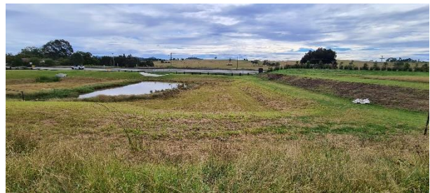
Photograph 12: Near BH1610 (Lot 1619), facing north. Showing existing basin and overflow area located in the northeast corner of site.
