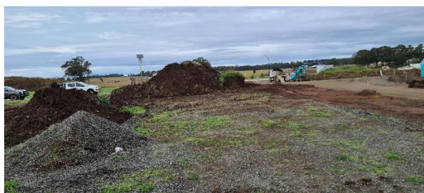
Photograph 1: From near BH1502 (Lot 1503), facing south.
