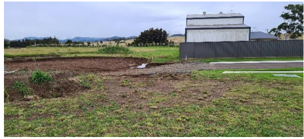
Photograph 8: Near BH1601 (Lot 1601), facing north.
