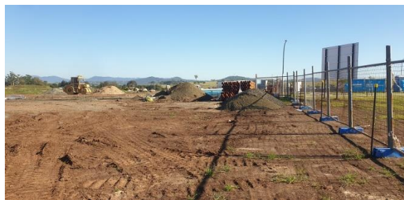
Photograph 12: From south-eastern corner of Lot 1423, facing north.
