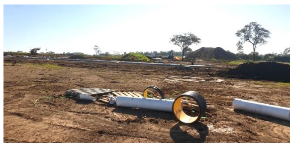
Photograph 10: From near south-western corner of Lot 1414, facing east.
