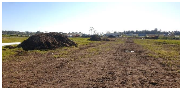
Photograph 6: From northern boundary of Lot 1408, facing east.
