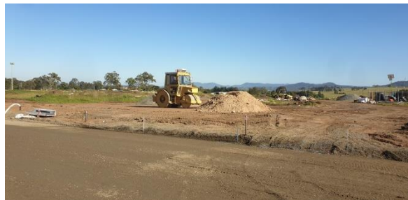
Photograph 14: From north-western corner of Lot 1423, facing northwest.
