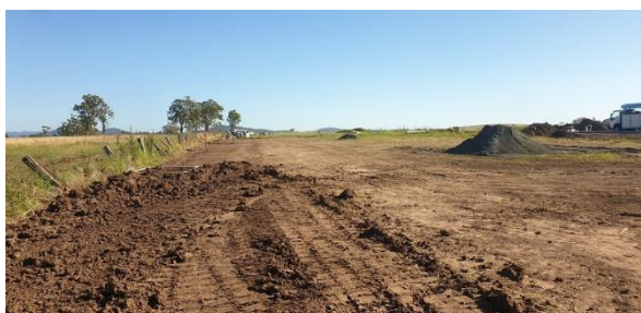
Photograph 9: From near south-western corner of Lot 1414, facing north.
