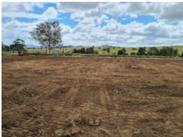
Photograph 11: Facing north from near BH113 near the centre of the site.
