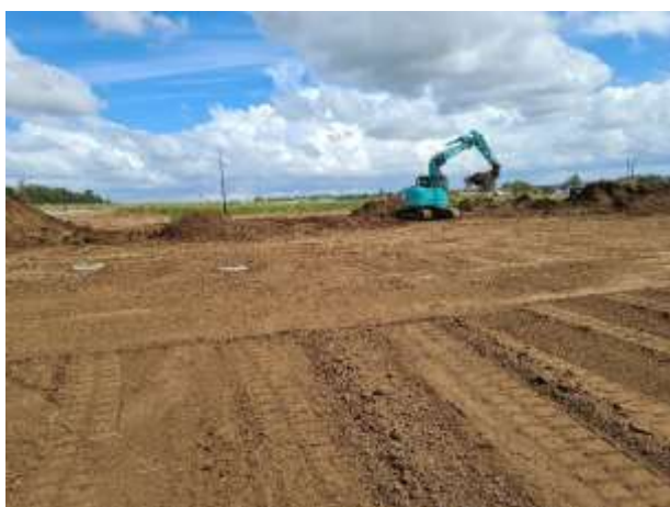
Photograph 13: Facing southwest from near BH111 near the centre of Stage 1.
