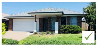
**PORTICO** - the façade addressing the street is to contain a covered portico which clearly defines the dwelling entry. The portico is to be a minimum of 25% of the width of the facade.
